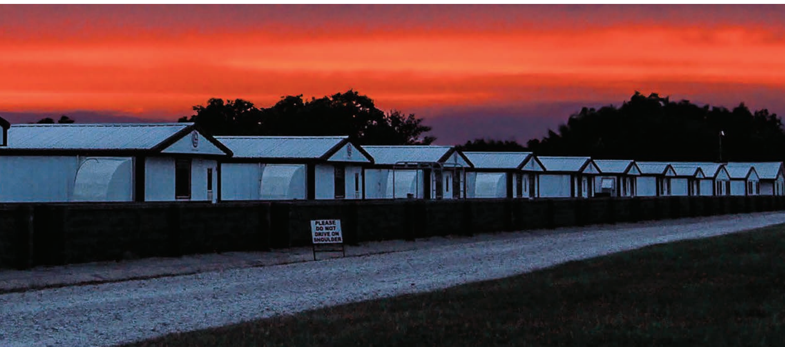
The Oklahoma State University Swine Research and Education Center, built in 2004, houses roughly 1,000 pigs. Photo by Justin Leonard.
